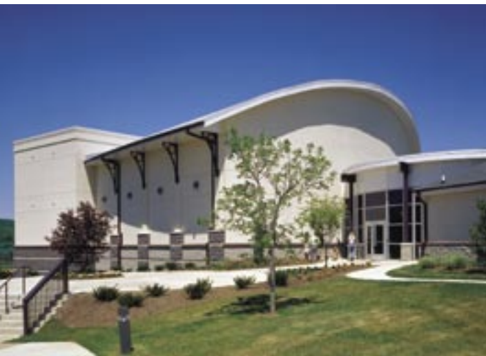
Highland School Center for the Arts, THE PLAINS, VA
